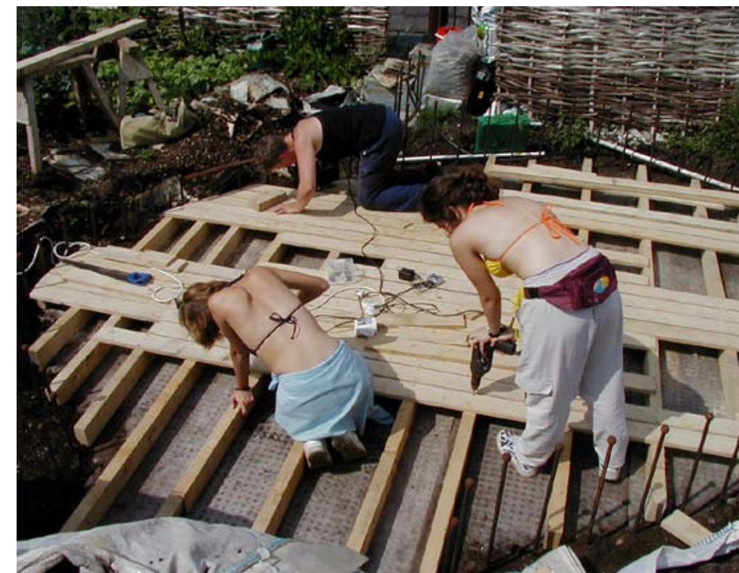
8. BUILDING THE ROOF DECK
