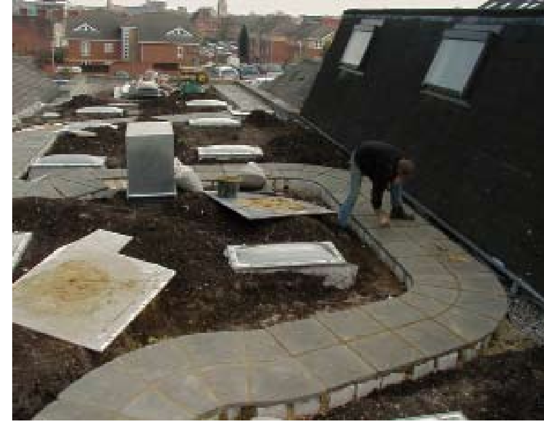
6. BUILDING THE PATHWAY
