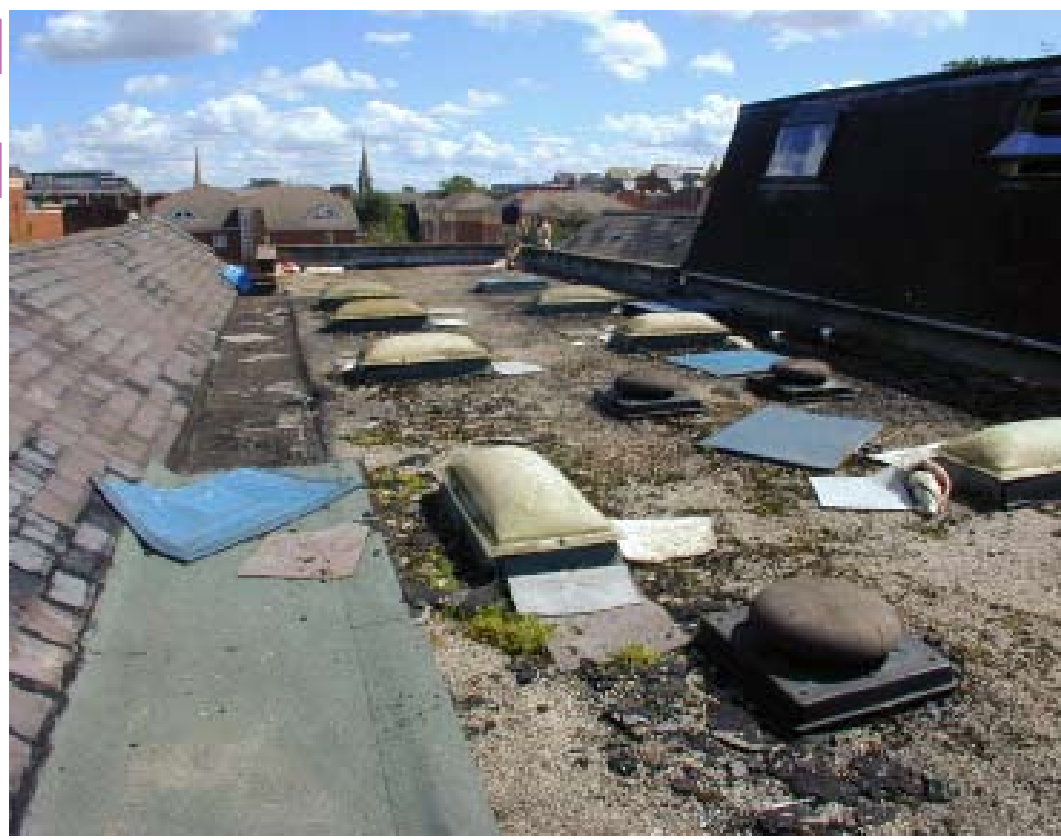
1. THE ROOF BEFORE CONSTRUCTION
