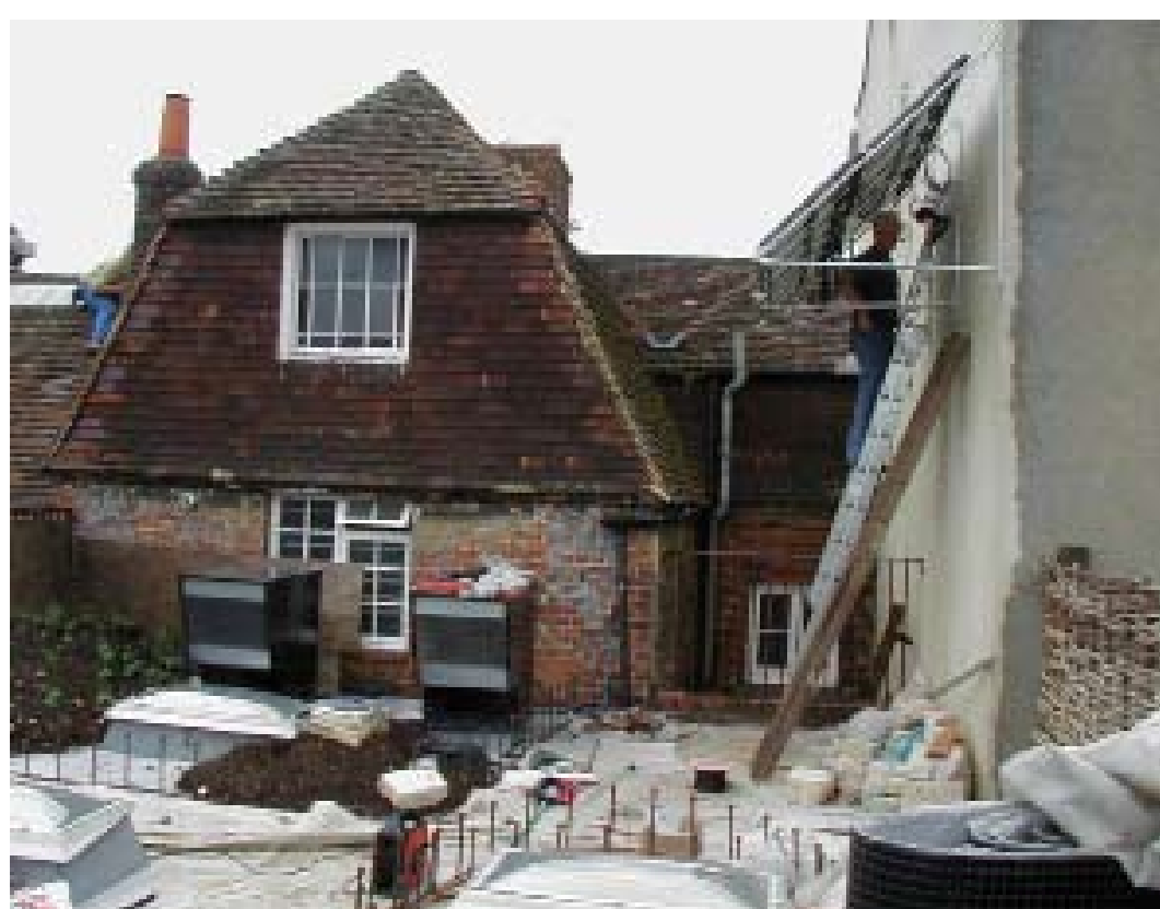
4. PUTTING UP THE SOLAR PANELS
