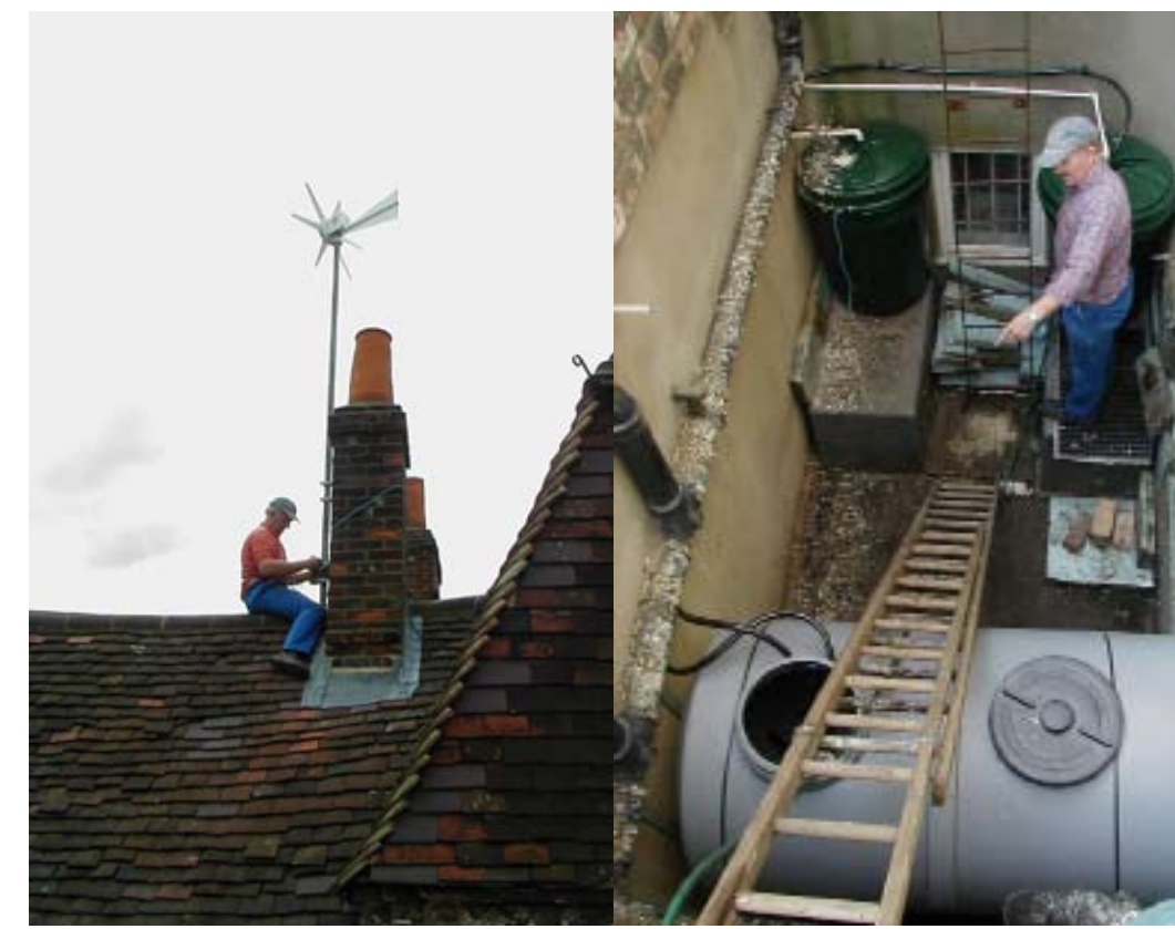
10. PUTTING UP A SMALL WIND TURBINE (LEFT) AND LOCATING THE TANK TO STORE RAINWATER (RIGHT)
