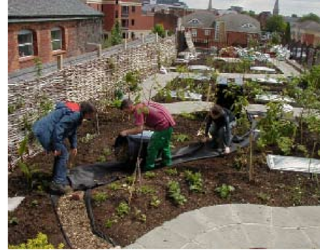
11. LAYING WOODCHIPS FOR ANOTHER PATHWAY AFTER PLANTING
