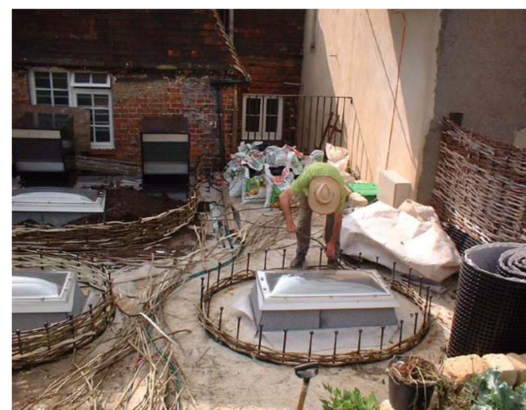
9. BUILDING THE BARRIER AROUND THE SKYLIGHTS
