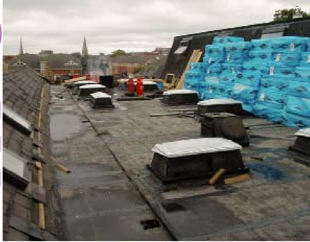
2. SEALING AND WATERPROOFING THE ROOF
